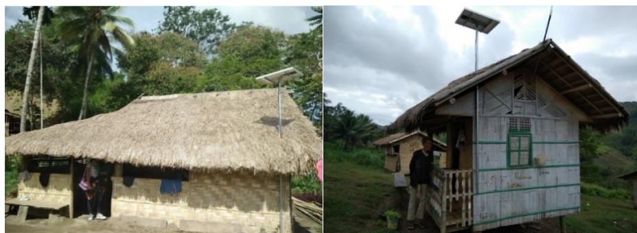
Diagram 8 : Roof-through Pole mounted installations on thatched roof
