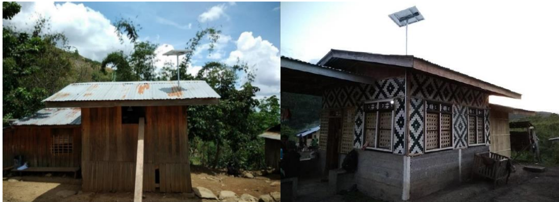
Diagram 7 : Roof-through Pole mounted installations on GI roofs
